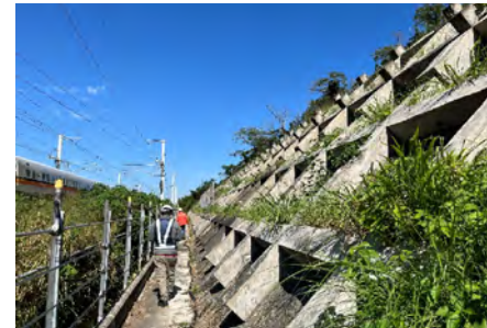
Entrust a technician to conduct a field survey on the slope
