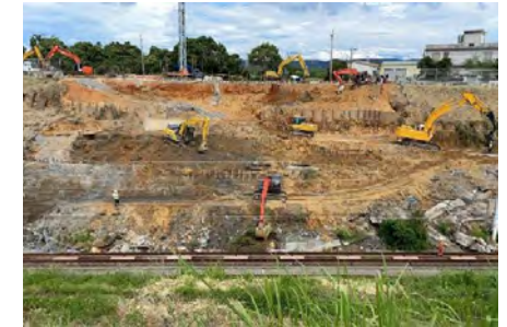
THSRC maintenance personnel performed on-site emergency repair works
