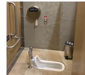
Install handrails in squatting toilets at railway stations
