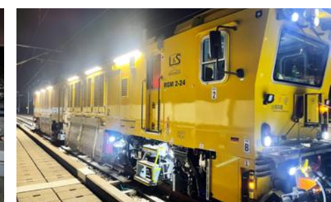
2023 Maintenance - Rail grinding
