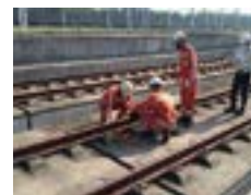
Rail Emergency Fishtail Sheet Installation Competition
