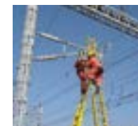
Colleagues from the Track & Power Department replaced the trolley arm of the overhead catenary system
