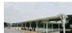
Add a rain shield from Exit 3 of Chiayi Station to the temporary parking area of Baotie 5th Road
