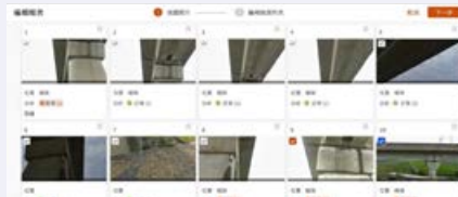
Inspection reports are automatically generated to support digitalized operations management.
