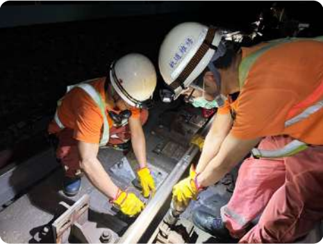
2025 Maintenance - Night-Time Track Maintenance
