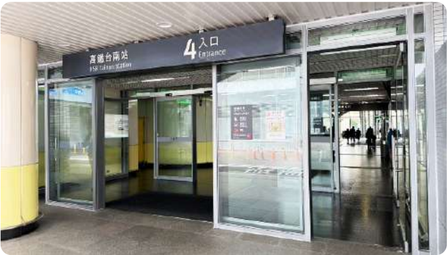
Completed the automation of No. 1 and 4 entrance doors at Chiayi and Tainan Stations in 2025.
