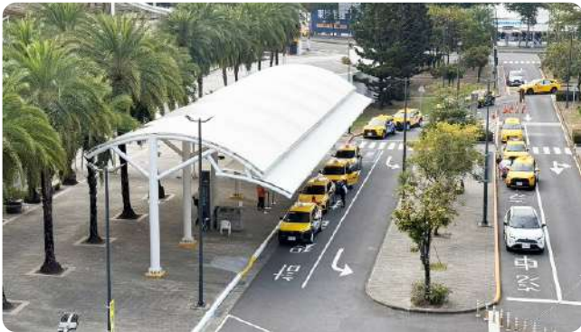
Completed the improvements to the rain shelters in the taxi queuing areas at Tainan Station in 2025.
