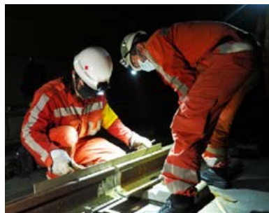
2024 Maintenance - night-time track maintenance
