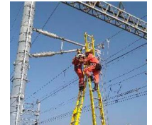
Colleagues from the Track & Power Department replaced the trolley arm of the overhead catenary system
