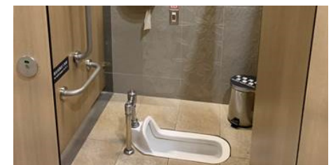
Install handrails in squatting toilets at railway stations
