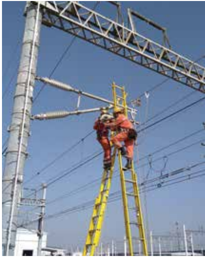
Track electrification unit colleagues change electric traction line rods
